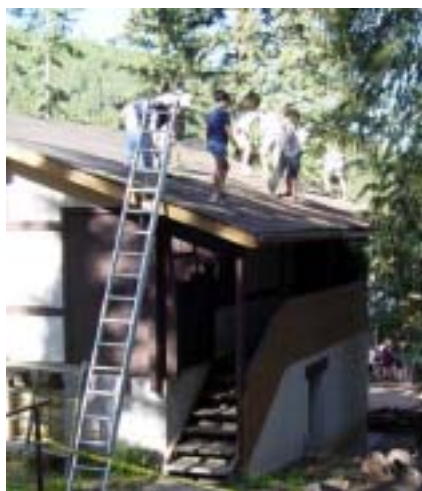
Eiger receiving a new roof this summer
