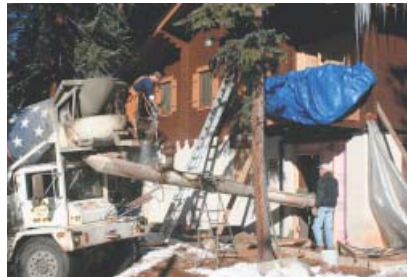
Leon Stutzman helps direct concrete into the Eiger Bathhouse
